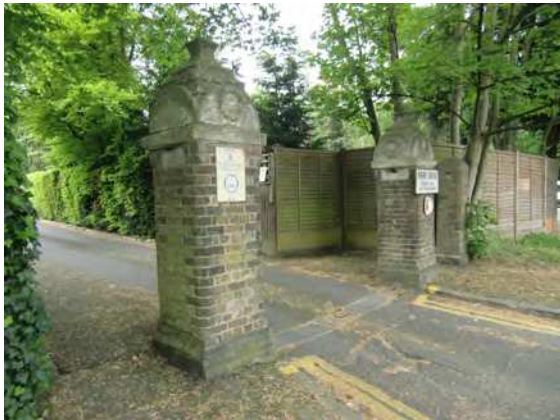
Picture 1.45 Late 19th century pillars to the former carriage driveway, now Park Drive
