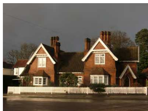
Picture 1.48 148 and 150 Uxbridge Road (former Gamekeeper's lodge)
