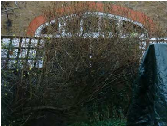
Picture 1.28 Central gauged red brick arch
