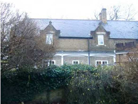
Picture 1.25 Three arches mark where the coach house doors were
