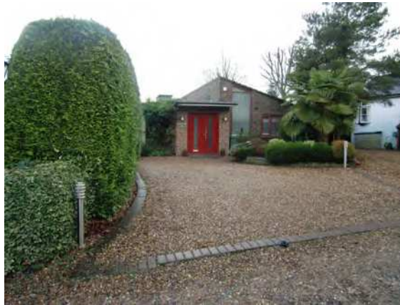
Picture 1.49 44a West Drive
