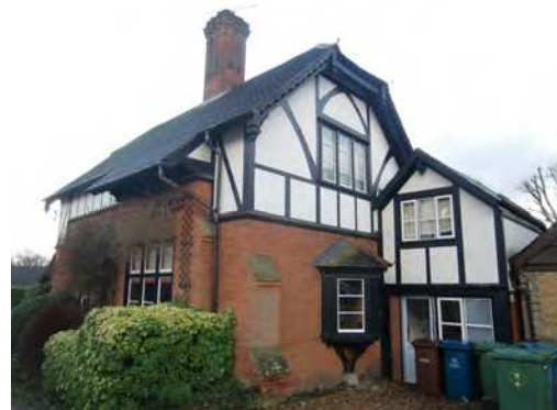
Picture 1.35 View looking south towards 47 West Drive
