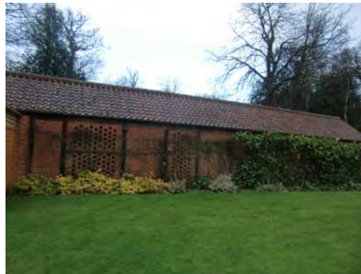
Picture 1.34 Replica drying sheds within the Kiln site, Brookshill re-using original clay pantiles
